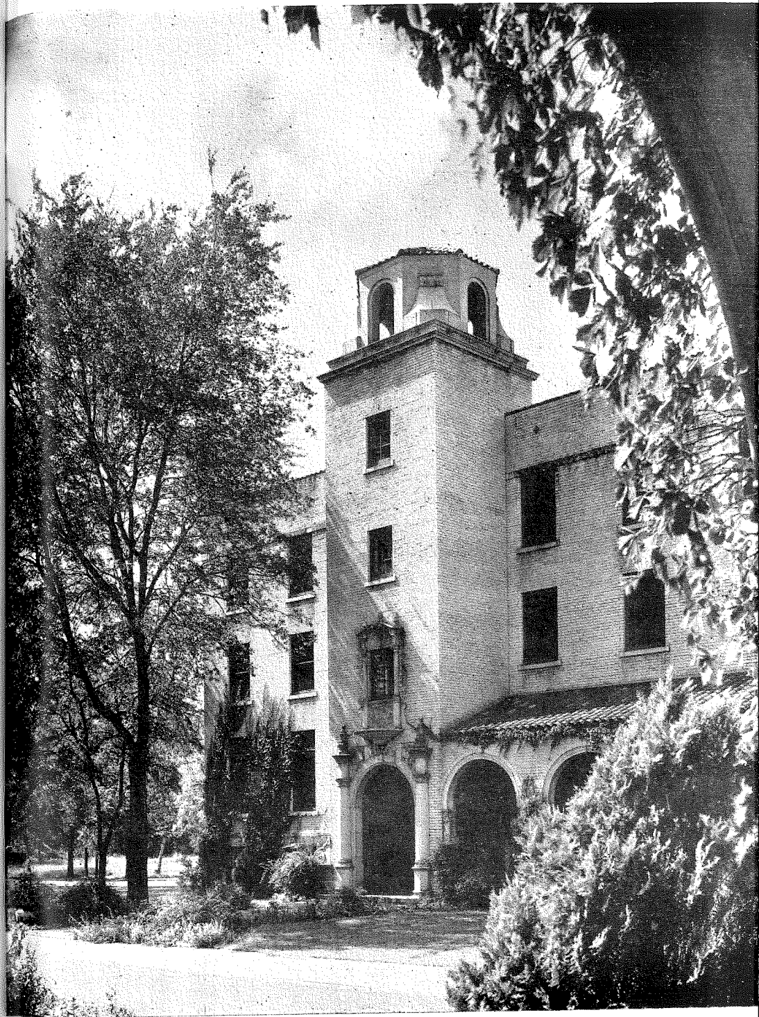
STEARNS HALL, DORMITORY FOR SINGLE MEN
